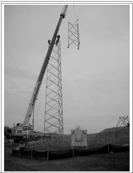
The new communications tower at 22<sup>nd</sup> Street rose rapidly on May 2<sup>nd</sup>. A crane lifted the sections into place as workers waited to bolt them together. In a matter of a couple hours the whole thing was up. The new tower will replace the old, skinnier, and slightly taller tower, which will be removed, with all its guy wires and anchors.
