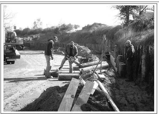
With Ron Holman Excavating doing the trenching and backfilling, Park Point volunteers construct a vertical post wall around the parking lot at 12<sup>th</sup> Street.
